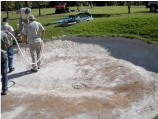
Sand flashing during 2 nd coat
