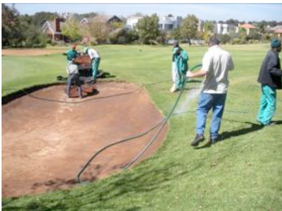
Final re-shaping of entry point
