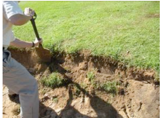
Re-shaping of entry point
