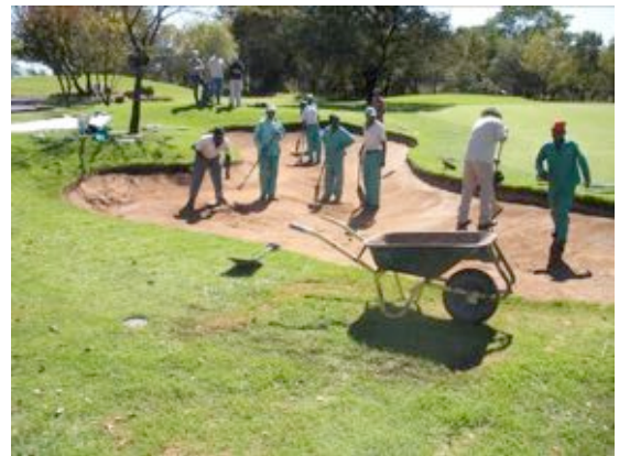
Sweeping and removal of loose gravel
