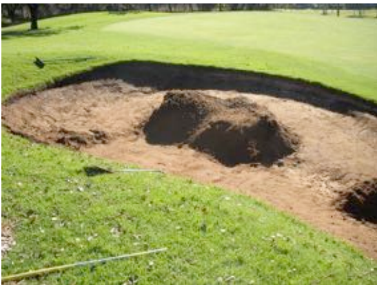
Removal of existing sand
