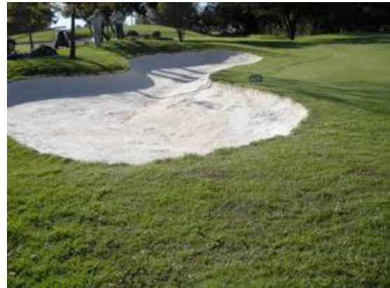
after 2 nd coat of Bunkertac™ and sand
