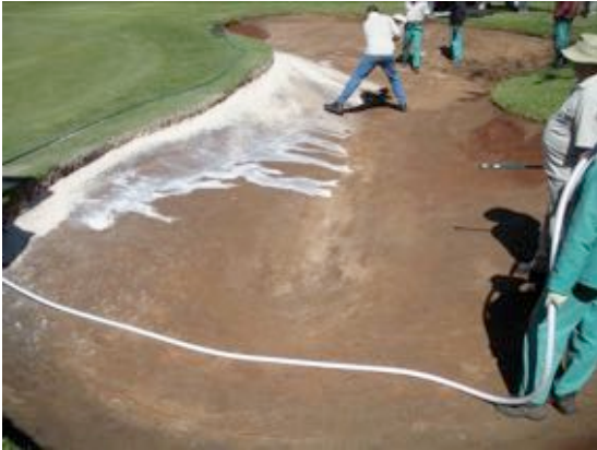
Sand placement 1st coat of Bunkertac™
