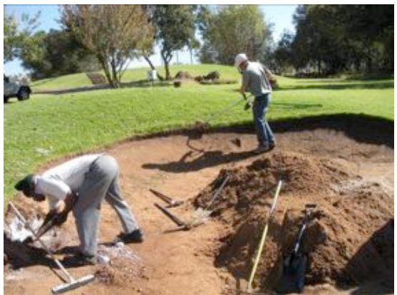
Trimming of edge and root removal
