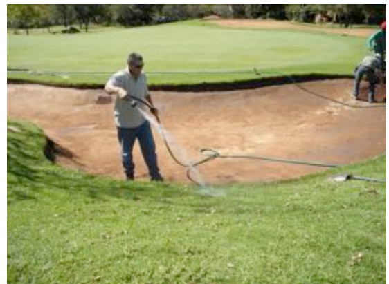
Pre-wetting to loosen tension of soil
