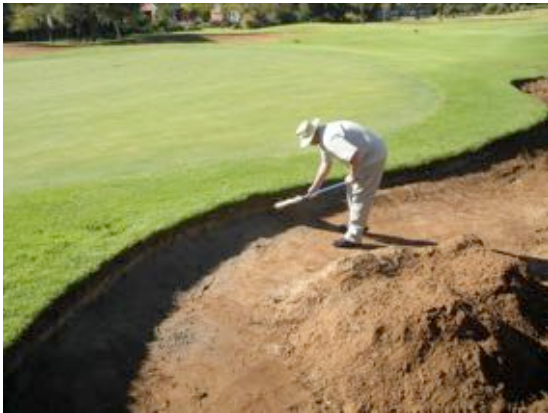
Sweeping of edge to remove loose sand
