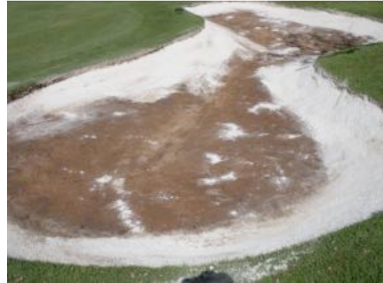
after 1 st coat of Bunkertac™ and sand
