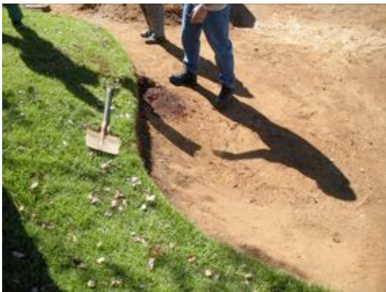
Topsoil filling after rock removal
