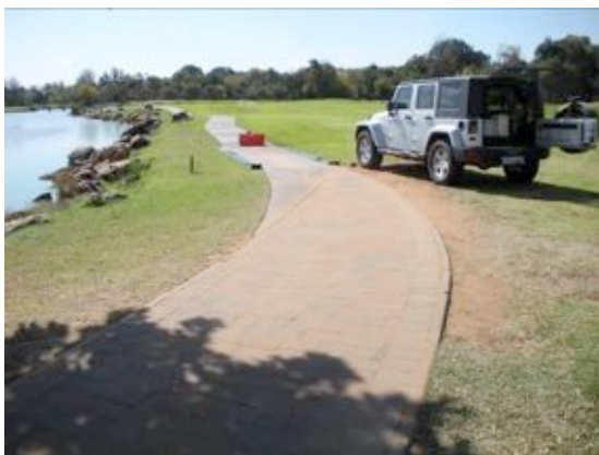
Preparation of paving block section
