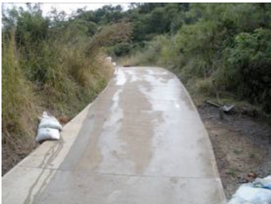
Ordinary concrete cart path
