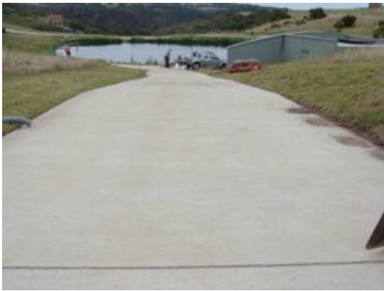
Ordinary concrete cart path
