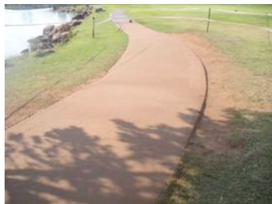
Damaged area repaired and covered
