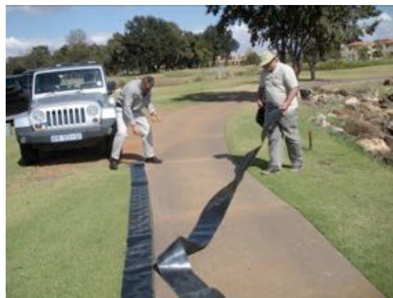
Placing of edging to protect grass
