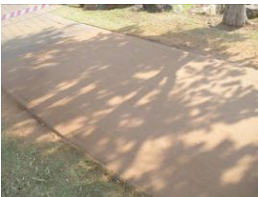
Damaged area repaired and covered
