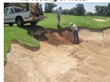
Repair of erosion problem
