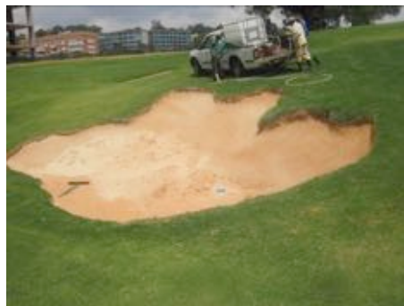
During Bunkertac Application
