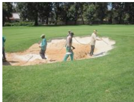
During Bunkertac Application
