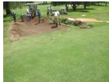
Re-routing of water
