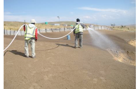
Hydrotac application at Nondela
