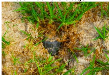
Sprinkler removal from edge
