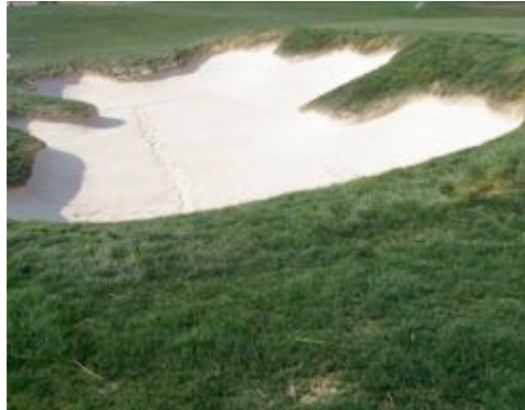
Bunker 3 after 1 st coat of Bunkertac™
