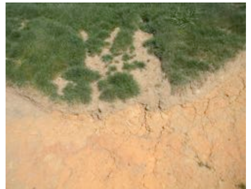
Collapsing edge and contamination source
