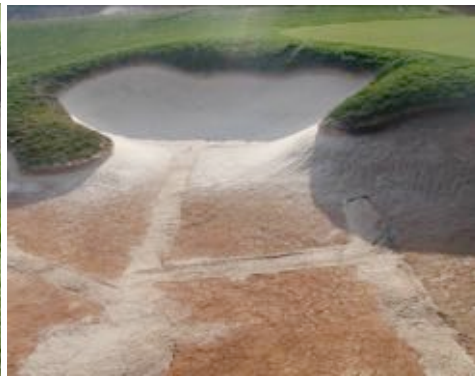
Bunker 1 during 1 st coat of Bunkertac™
