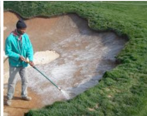
Bunker 2 during pre-coat of Bunkertac™
