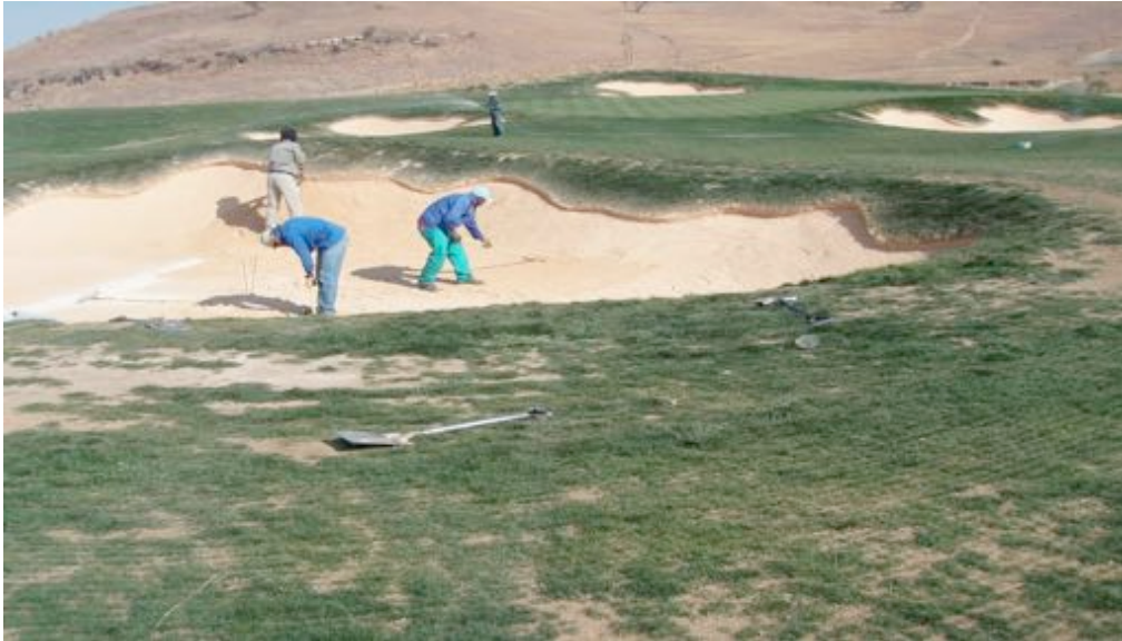
Installation of sand after Bunkertac™ application
