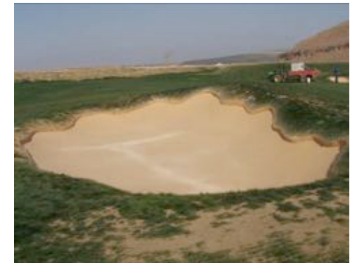
Bunker 4 after 6 th coat of Bunkertac™
