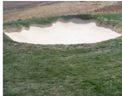
Bunker 4 after 3 rd coat of Bunkertac™
