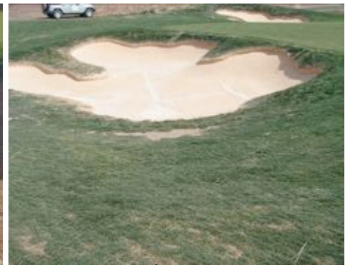
Bunker 1 after 6 th coat of Bunkertac™
