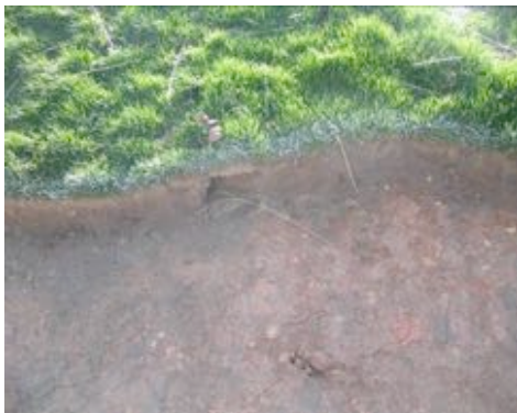
Hole in the edge needing to be filled
