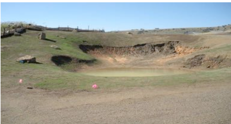
Hole 13 Hillside 1 Large Fairway Bunker prepared for repair
