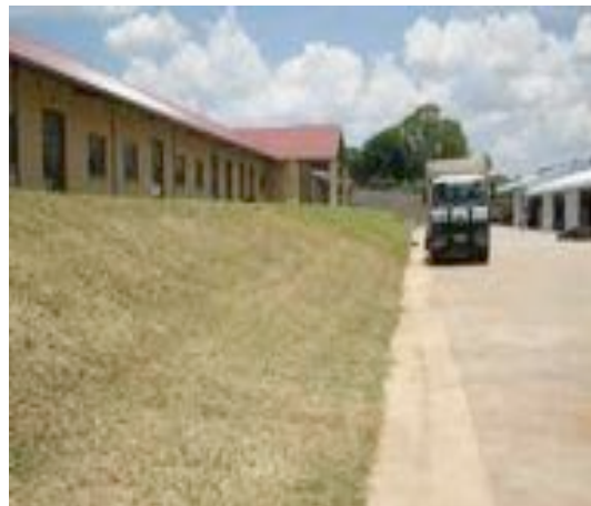
Hillside After Hydrotac application
