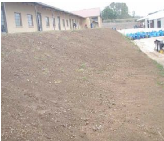
Hillside before Hydrotac application
