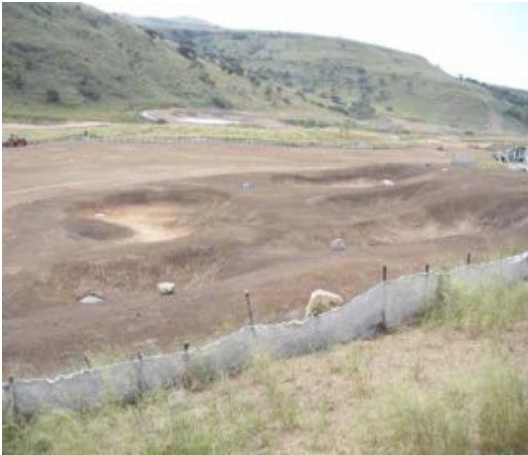
Nondela Hole 13 Before Application
