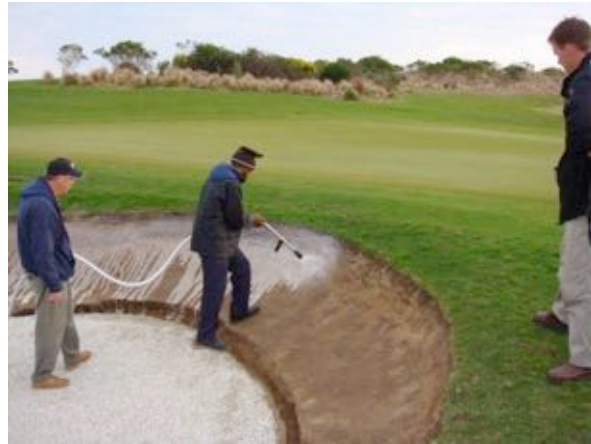
Ndiphiwe Melityala applying first coat to bunker
