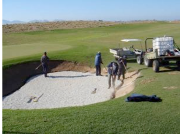
Sweeping of loose aggregate material
