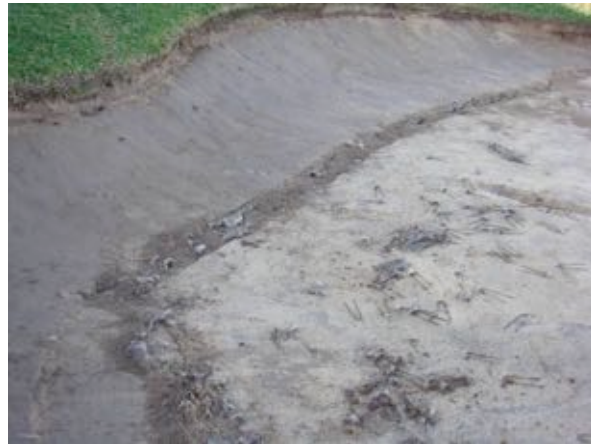
Removal of geo fabric and staples
