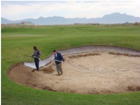
Application of first coat by Ndiphiwe Melityala
