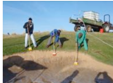
Brooms used for sand placement
