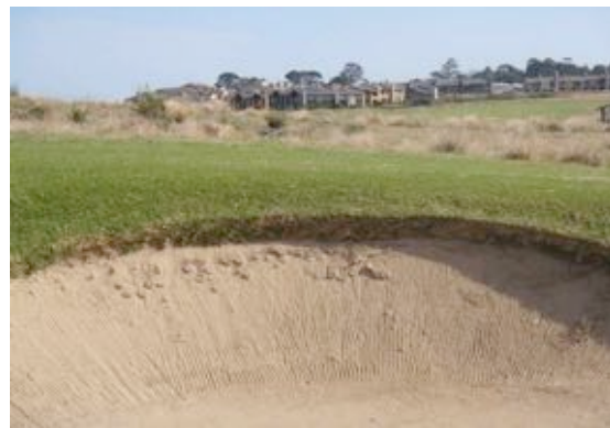
Exposed Geo Fabric on bunker faces and edges
