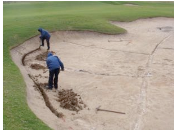
Digging of trench for shade cloth
