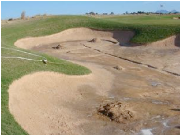
Bunker face following sand placement after 3 rd coat
