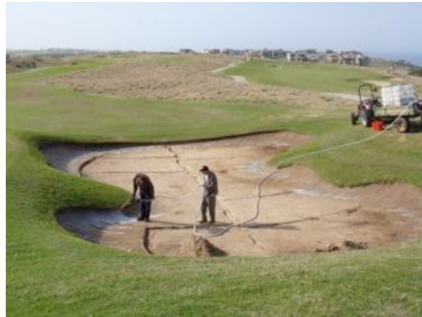
Bunker during application of second coat
