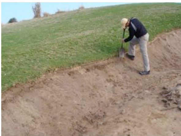
Repair of area where geo fabric was removed
