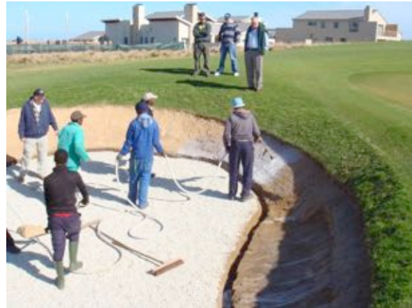
Sand placement during application of third coat
