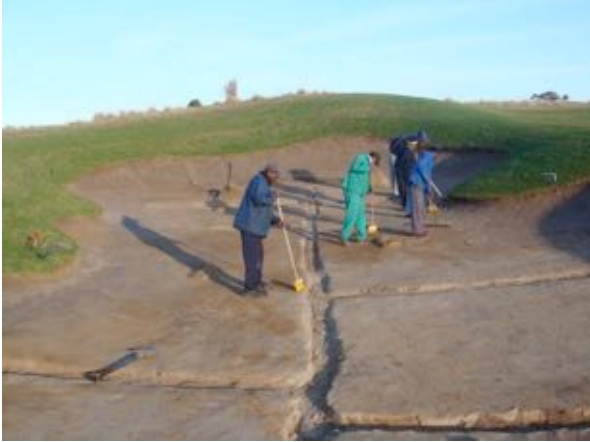
Sweeping of loose aggregate throughout bunker
