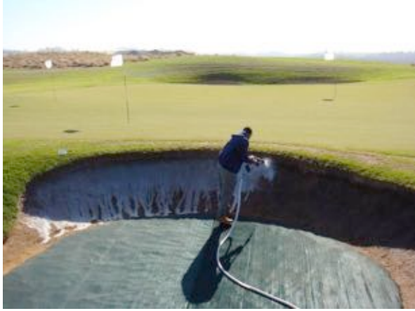
Application of first coat to practice bunker
