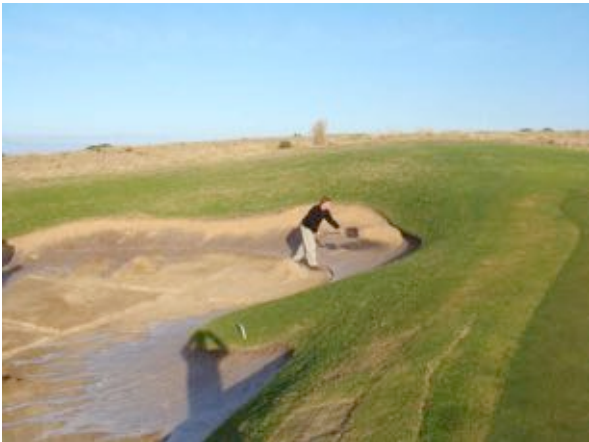
Placement of sand immediately after third coat
