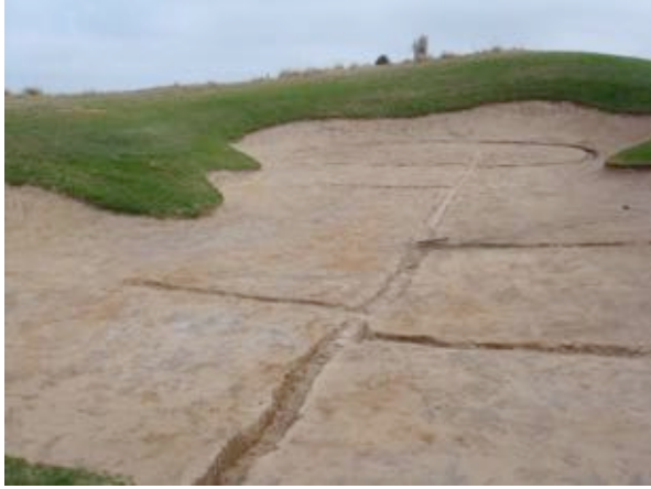
Repaired Drainage System
