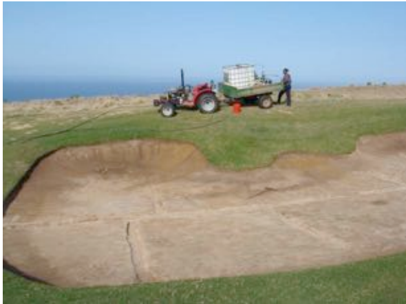
Bunker prepared for application
