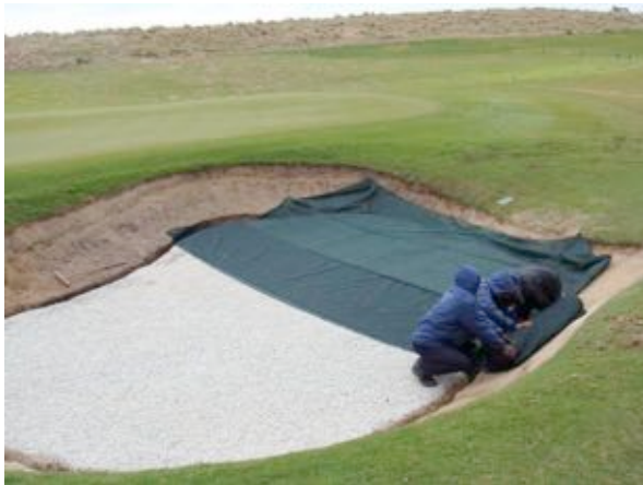
Placement of shade cloth over gravel base
