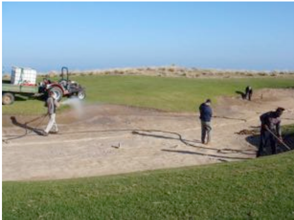
Slight moistening of the soil before application
