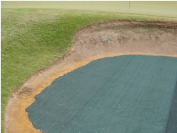
Properly prepared bunker for application
