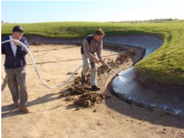
Charl Blaauw applying first coat to bunker
