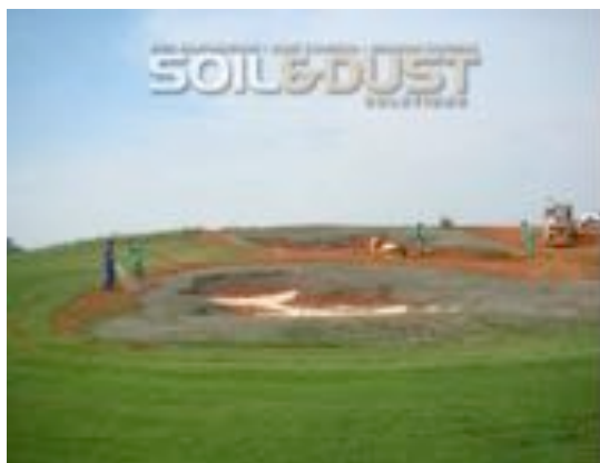
Hydro seed application Driving Range Bunker 2
