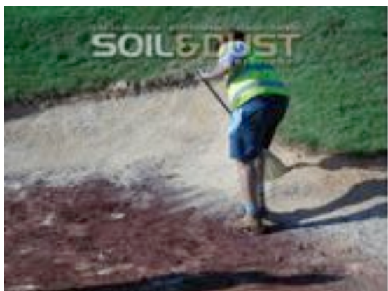
Placement of bunker sand using whisk broom
