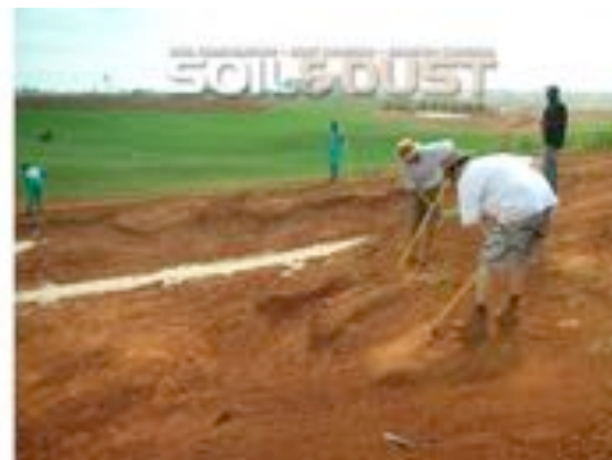
Preparation of Driving Range Bunker 1
