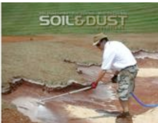
Bunkertac application to Driving Range Bunker 2
