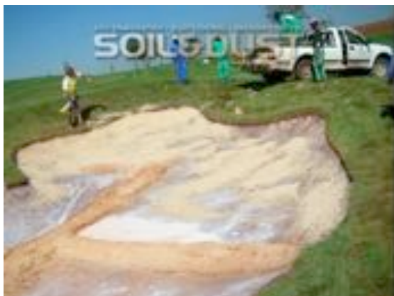
Placement of bunker sand after application
