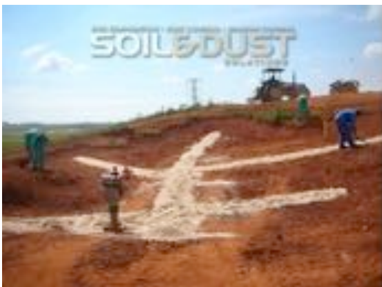
Driving Range Bunker 1 prior to hydro seeding
