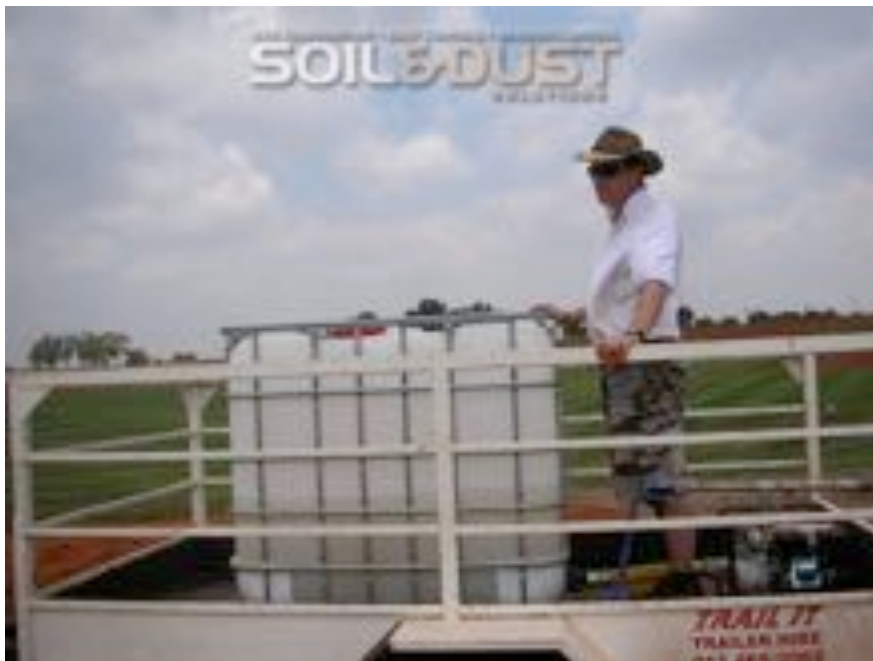
Hired Trailer showing tote used for Bunkertac mix and pump set up with T-fitting and return valves
