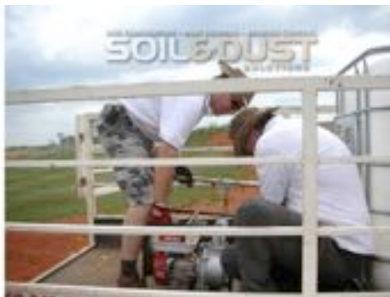
Preparation of pump for Bunkertac application
