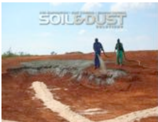
Hydro seed application Driving Range Bunker 1
