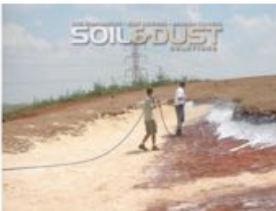
Bunkertac application over the bunker sand
