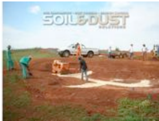
Compaction of Driving Range Bunker 2
