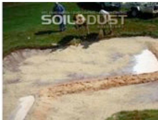
Sweeping bunker sand into steep faces of bunker
