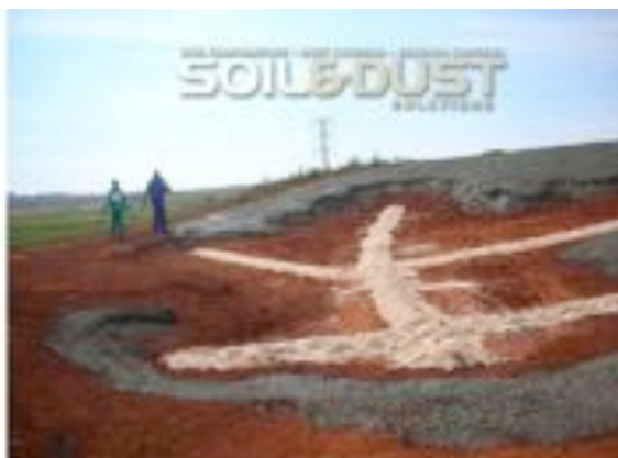
Hydro seed application Driving Range Bunker 1
