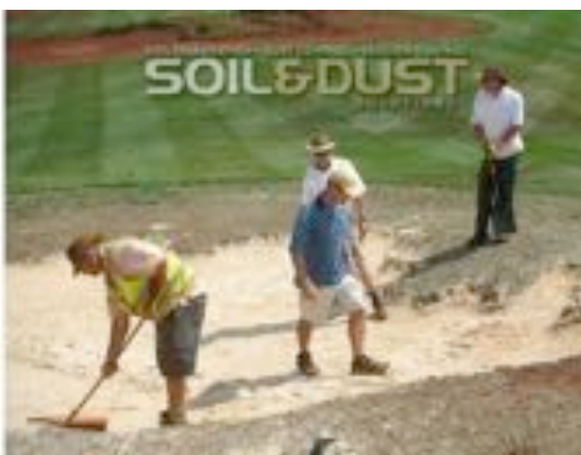
Sweeping bunker sand against steep faces
