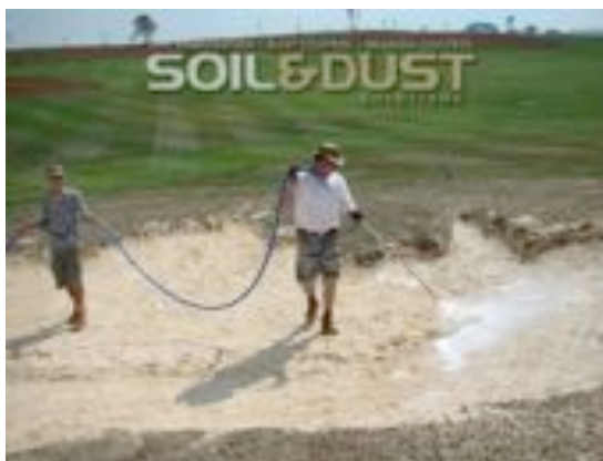
Bunkertac application to bunker sand
