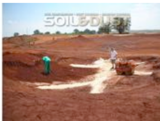
Preparation of Hole 1 Bunker 1
