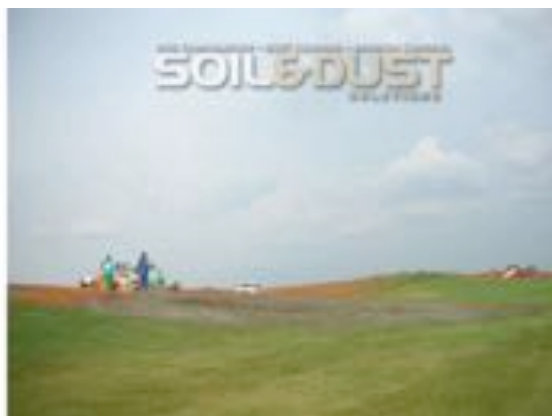
After Hydro seeding Driving Range Bunker 2
