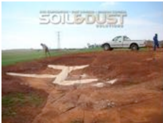
Driving Range Bunker 2 prior to hydro seeding
