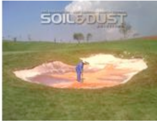
Hole 4 Bunker 3 after bunker sand placement
