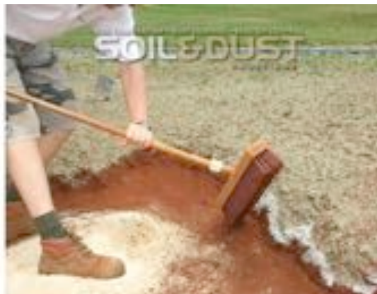
Sweeping of steep faces prior to application
