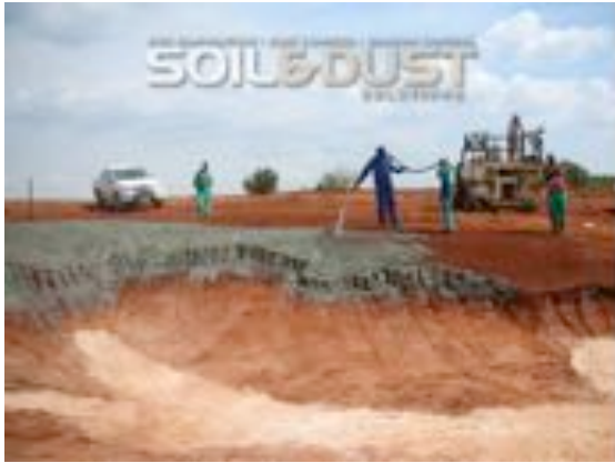
Application of hydro seed mix
