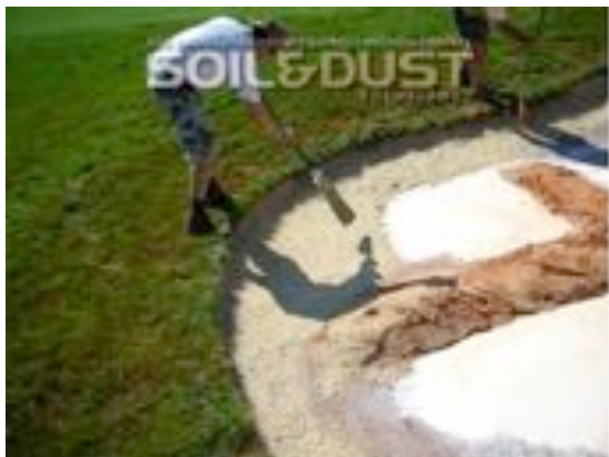
Whisk corn broom being used for sand placement Whisk corn broom being used for sand placement
