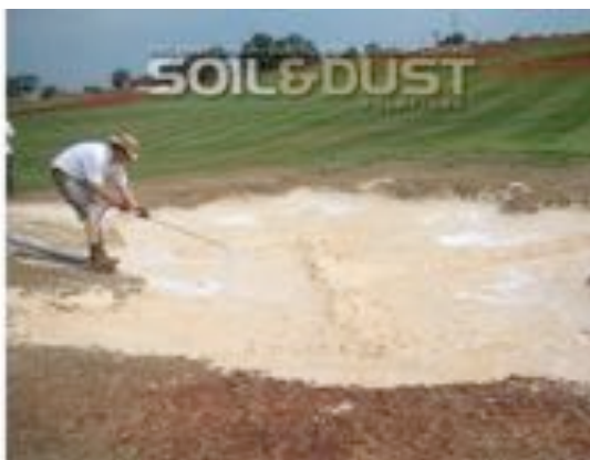
Bunkertac application to bunker sand
