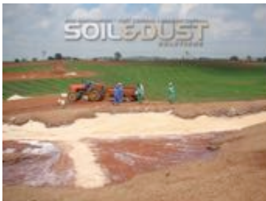
Bunker sand layer over half of bunker 1
