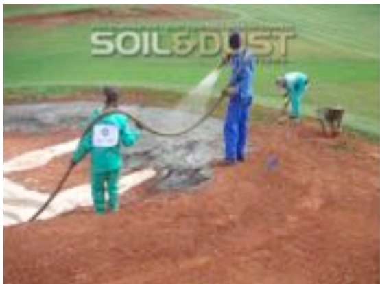
Hydro seed application Driving Range Bunker 2
