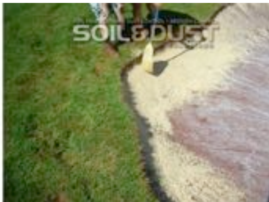
Whisk corn broom being used for sand placement Whisk corn broom being used for sand placement
