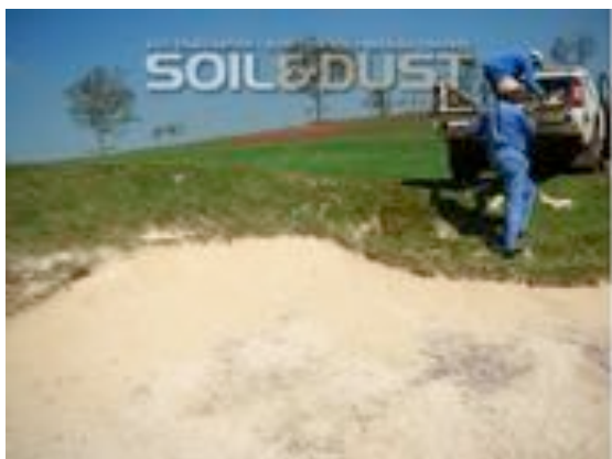
Bunker sand placement along steep face
