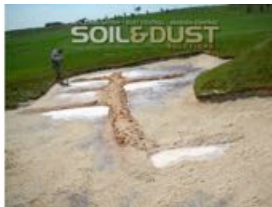
Hole 4 Bunker 3 after bunker sand placement
