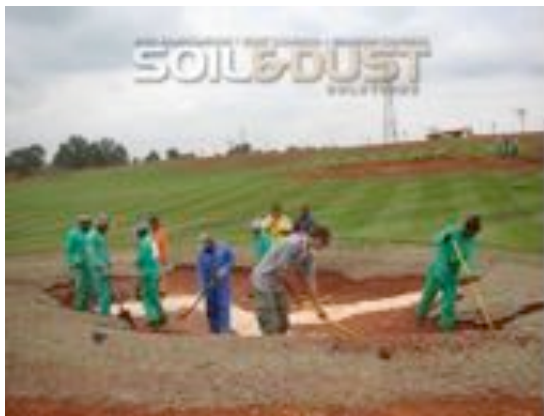
Preparation of Driving Range Bunker 2
