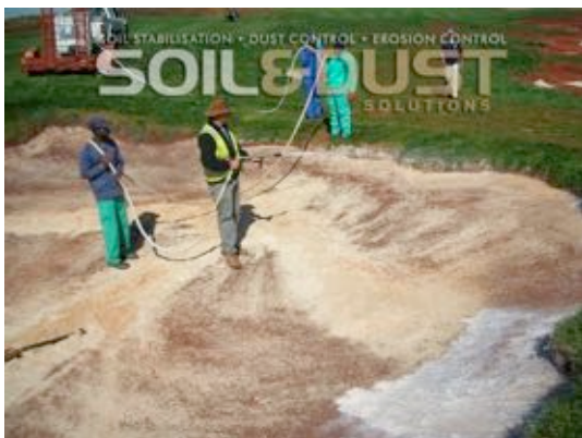
Bunker D during Bunkertac application
