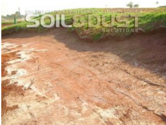
After first coat of Bunkertac to unsanded area
