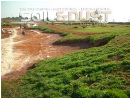
Waste Bunker Bunkertac area with no sand
