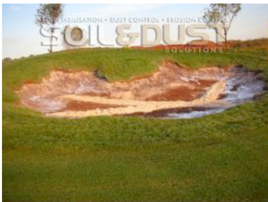
Bunker E during Bunkertac application
