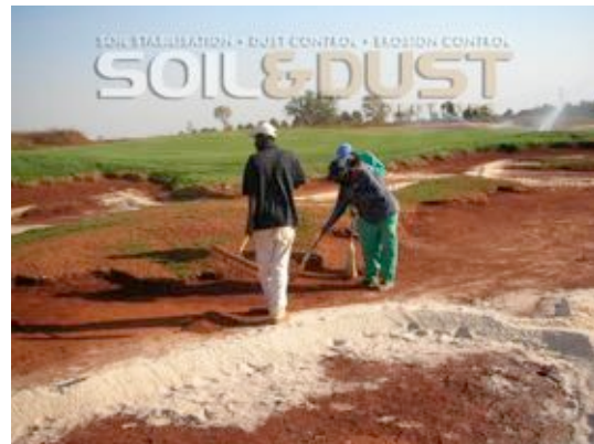
Preparation of Waste Bunker using brooms
