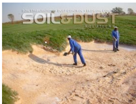
Bunker D sand placement after application
