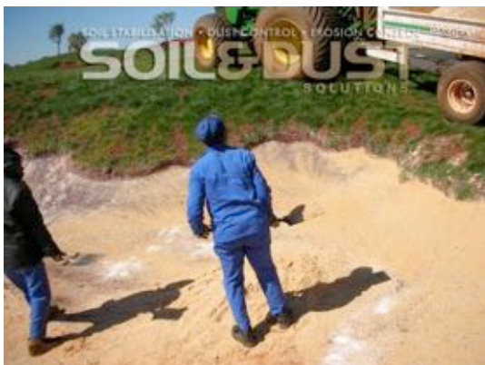
Bunker B sand placement after final coat
