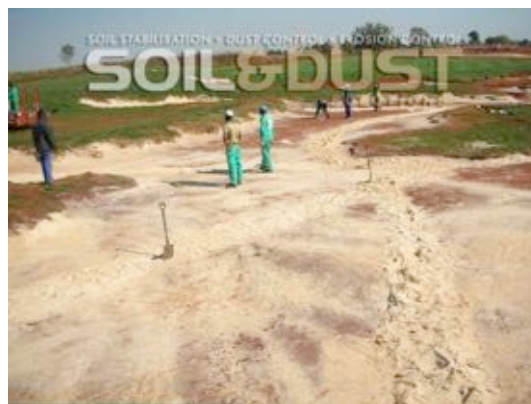
Waste Bunker showing placement of sand
