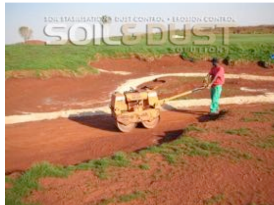
Compaction of area of Waste Bunker
