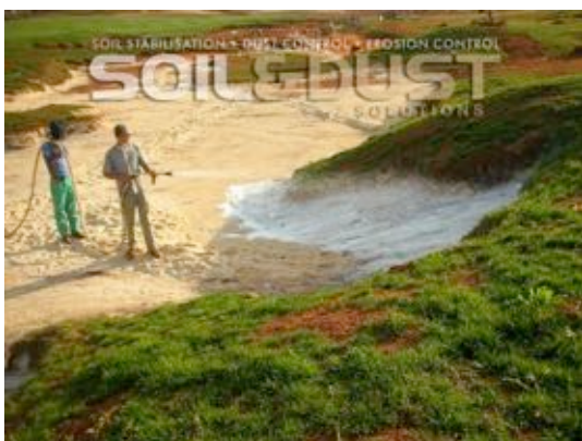
Waste Bunker during Bunkertac application
