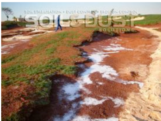
Waste Bunker following first coat of Bunkertac
