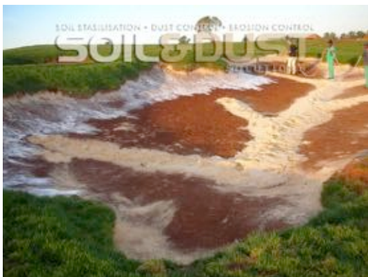
Bunker F during Bunkertac application
