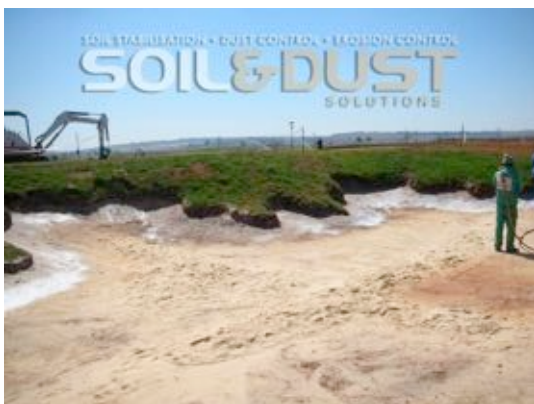
Waste Bunker during Bunkertac application
