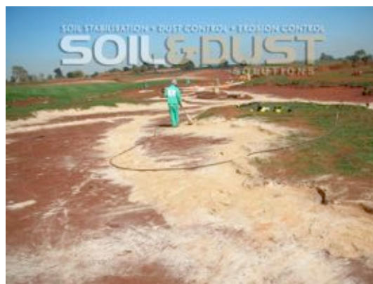
Waste Bunker sweeping of sand against edge
