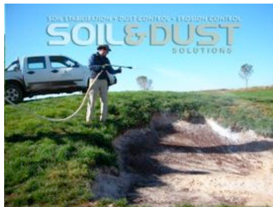
Bunker A during Bunkertac application
