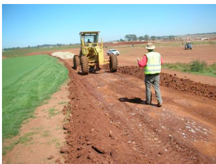
Grader used for prep and leveling
